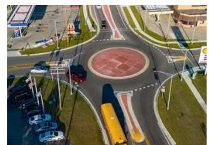
New roundabouts on the WIS54 project in Outagamie County
